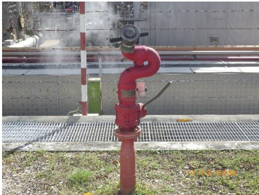
Fire Water Monitor with Foam Induction
